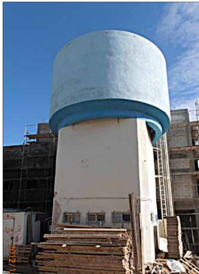
Brandeis tower during preservation.
