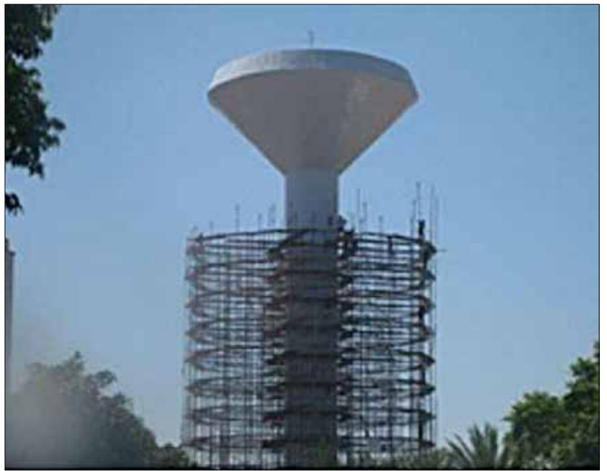
South Tower during application.
