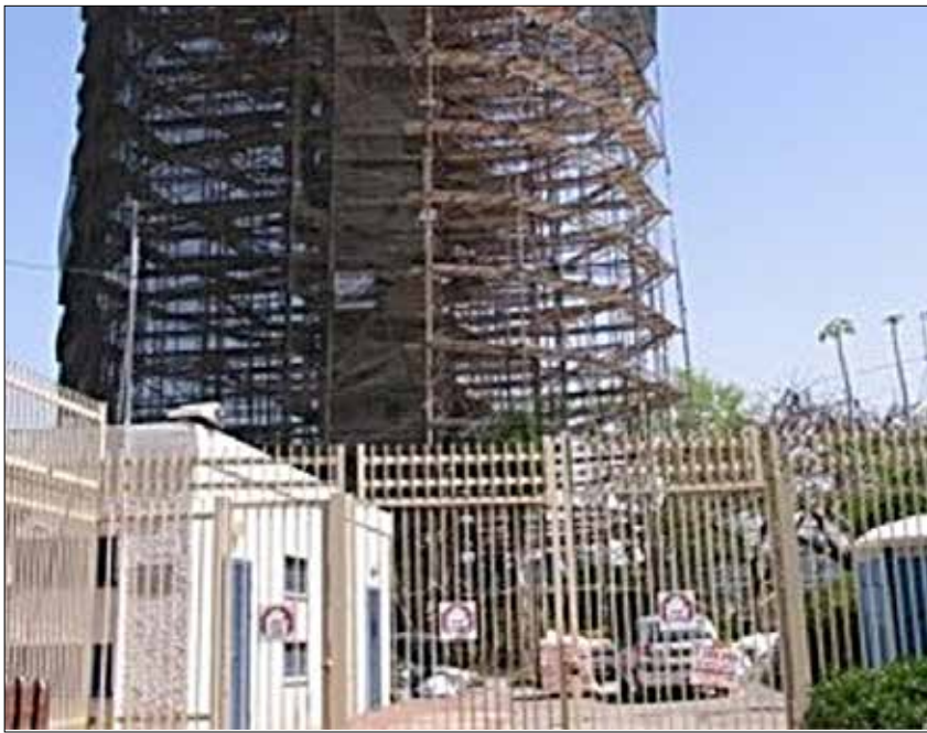
South Tower during application.
