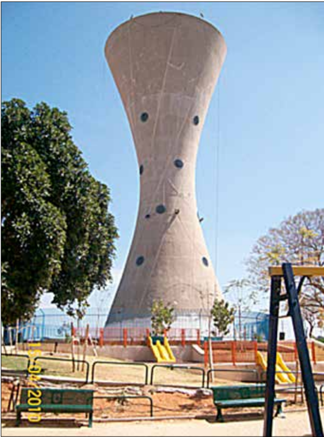
Tower prior to restoration
