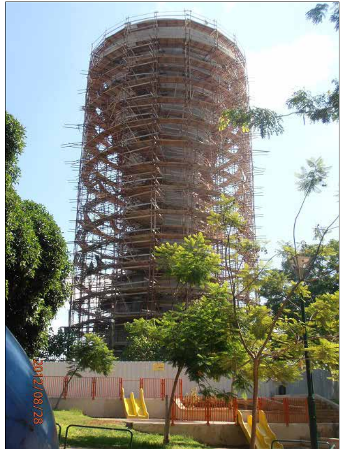
Tower during restoration
