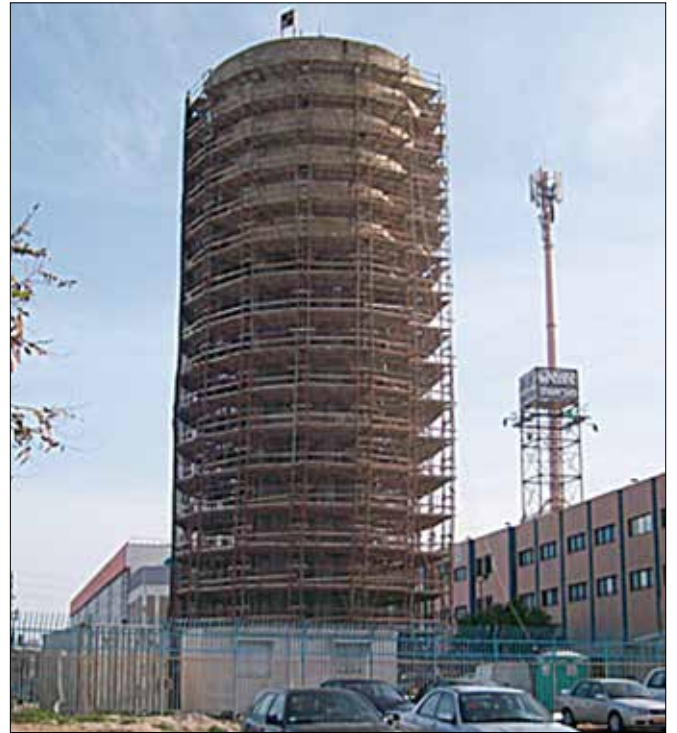
Holot Tower during restoration
